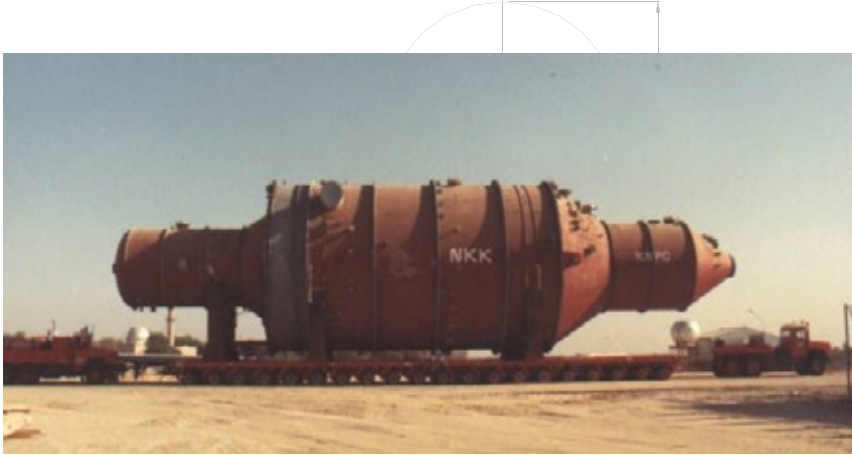
1984 - Transporting a 370 te reactor in the U.A.E.
