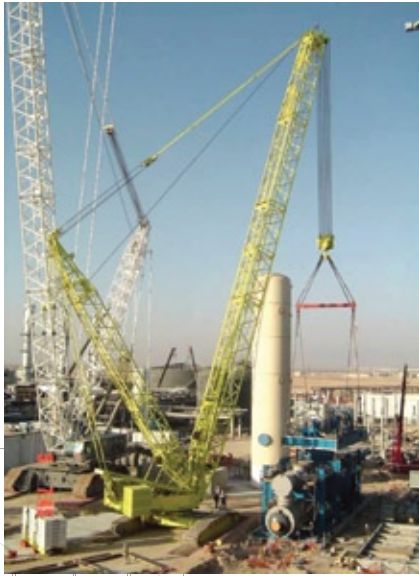
2004 - Lifting a 260 te compressor in Qatar.
