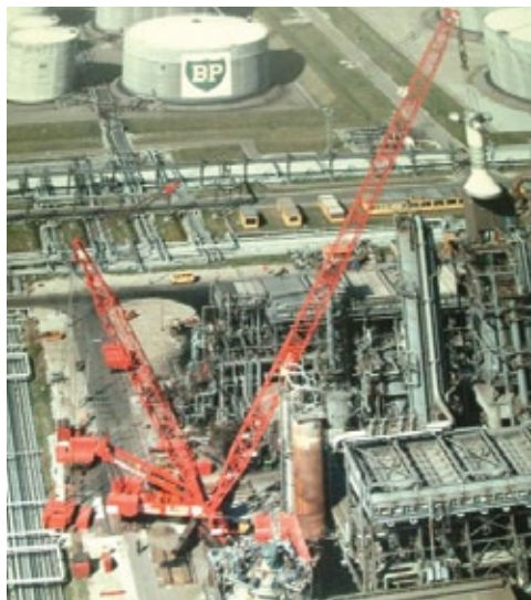
1988 - Lifting a 225 te reactor head in Holland.
