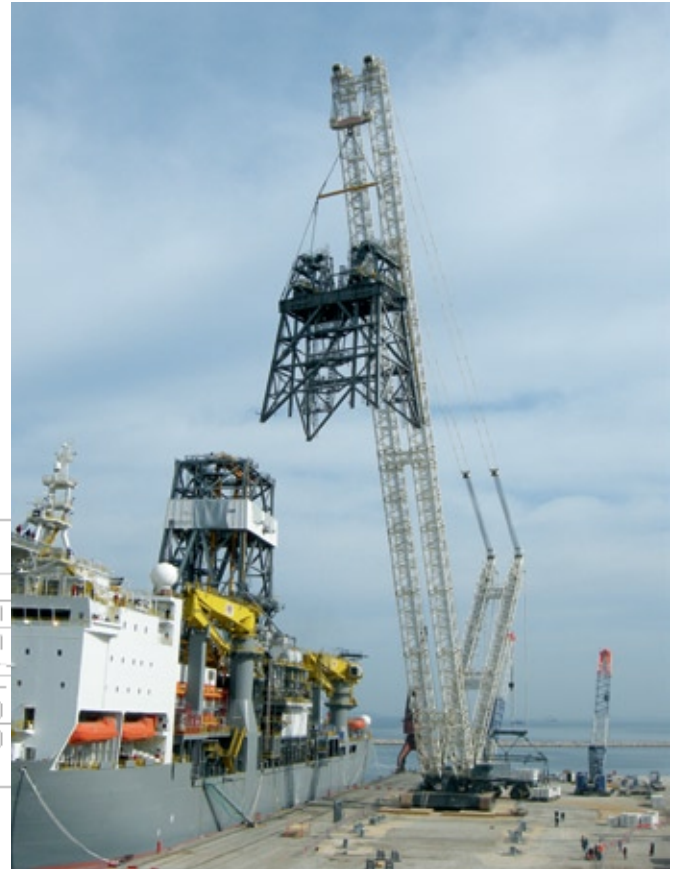
3,200te capacity Demag CC8800-1 with a crawler twin attachment lifting 548te at 46m radius with 138m boom in Europe.
