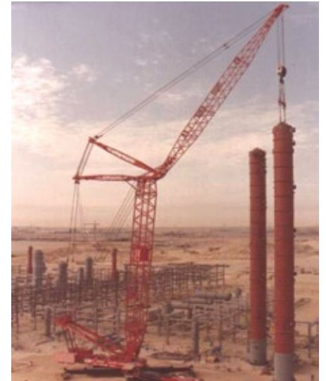
1992-Erecting a 200 te vessel in the K.S.A.
