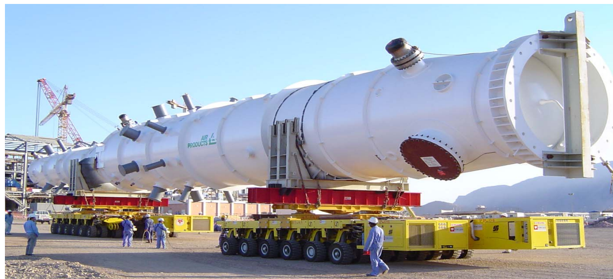
Transporting a 270 te cryogenic exchanger using 24lines SPMT in Oman.
