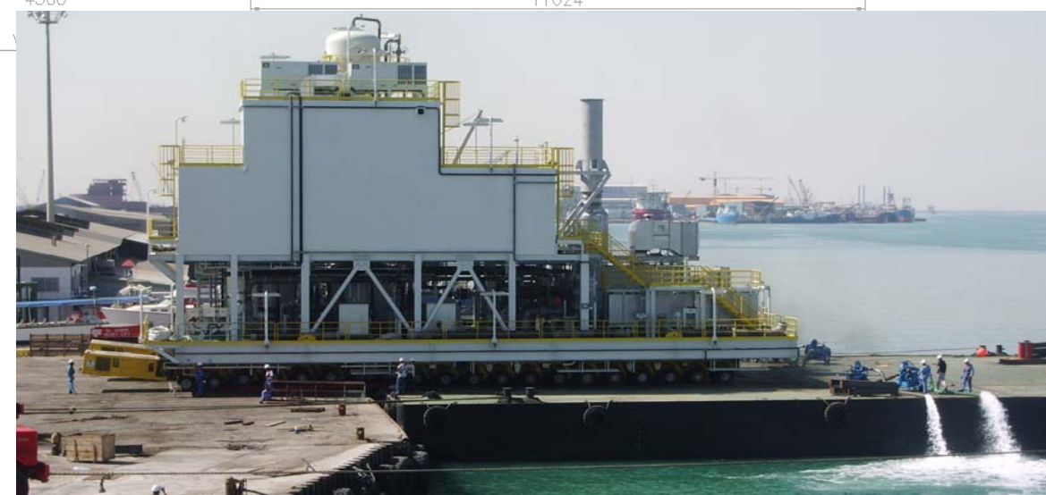
Load out a 550 te module at Al Jaber Mussafah jetty.
