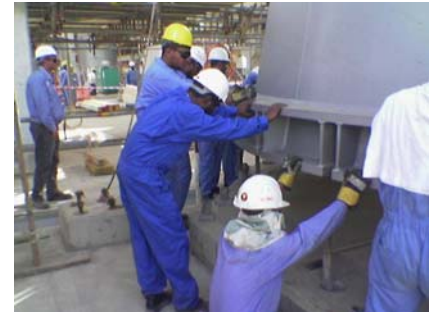
Our surveying team performs checks on foundation holding bolts and vessel orientation prior to lowering onto foundation.
