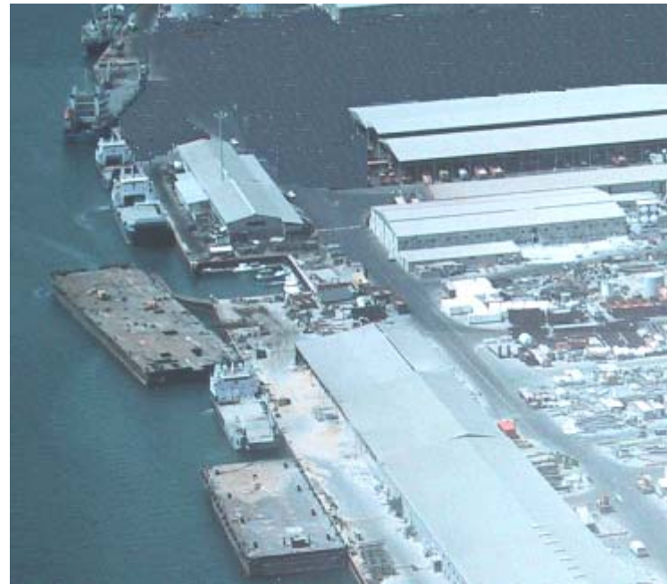
Al Jaber marine jetty facility
