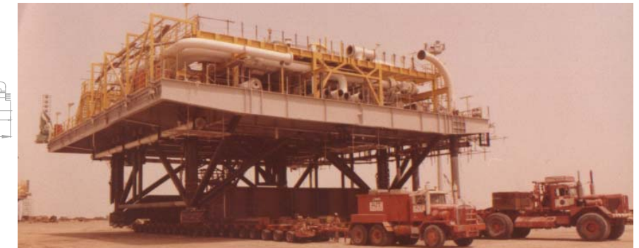
1985- Transporting & load out a 210 te offshore module in the U.A.E
