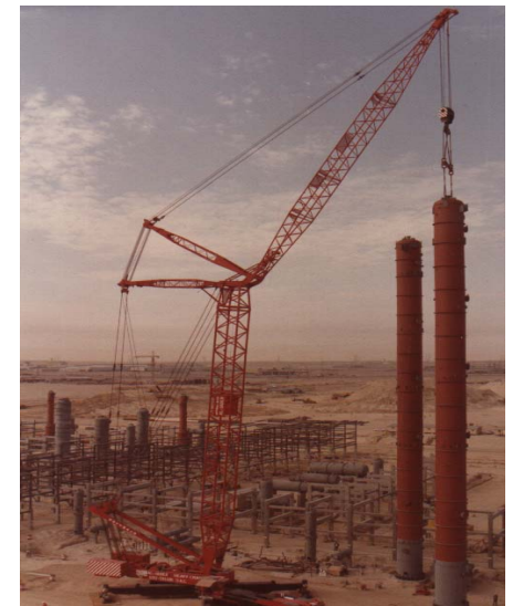
1992- Erecting a 200 te vessel in the K.S.A.
