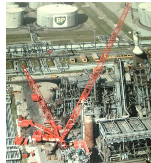
1988- Erecting a 225 te reactor head in Holland.
