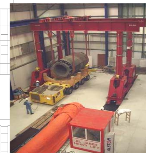
Handling a generator stator
