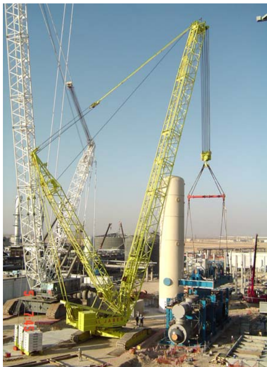
2004- Erecting a 260 te compressor in Qatar.
