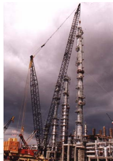
1986- Erecting a 210 te vessel in Iran.
