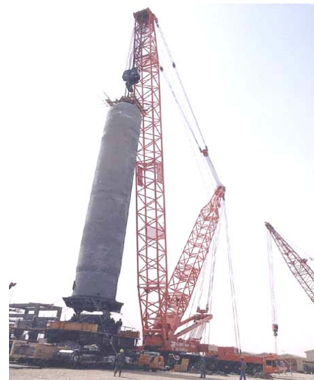
1985- Erecting a 833 te reactor in Kuwait.
