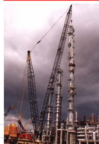
1986- Erecting a 210 te vessel in Iran.
