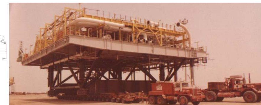
1985- Transporting & load out a 210 te offshore module in the U.A.E
