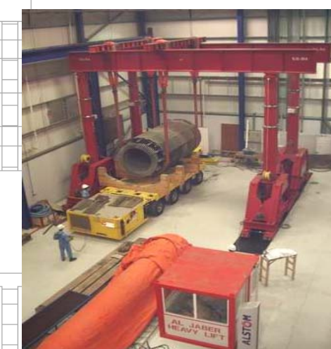
Handling a generator stator
