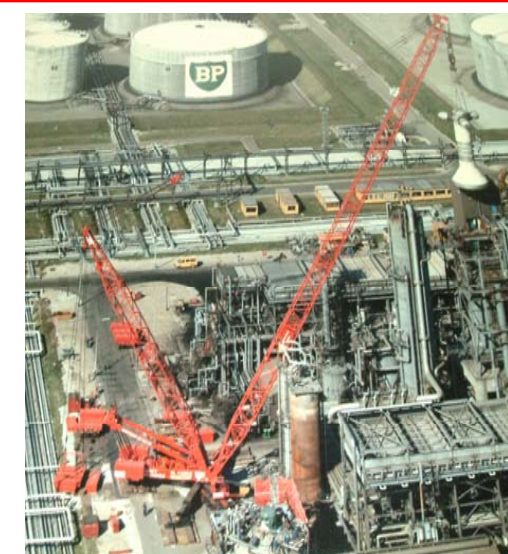
1988- Erecting a 225 te reactor head in Holland.
