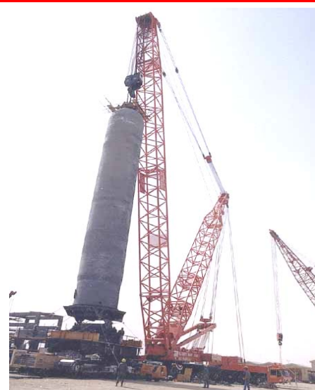
1985- Erecting a 833 te reactor in Kuwait.
