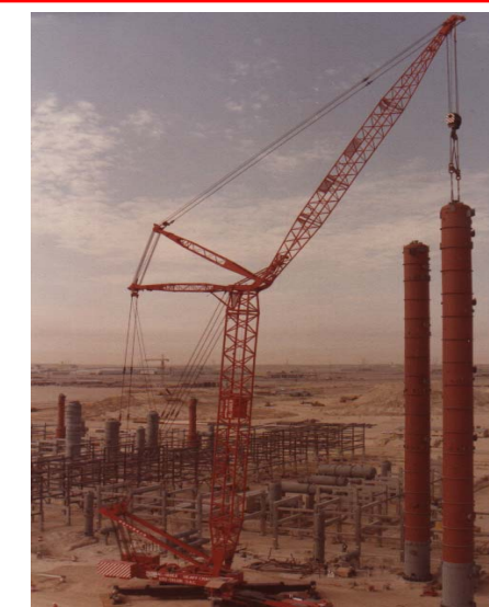
1992- Erecting a 200 te vessel in the K.S.A.
