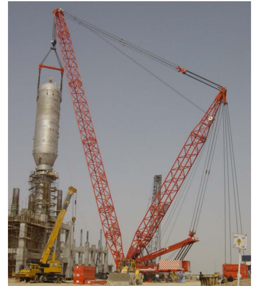
Erecting a 360 te demethanizer in Iran at 30m above ground level in Iran.
