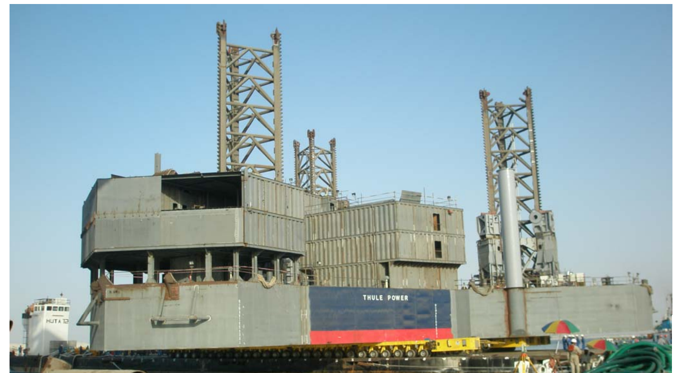
Weighing a 4015 te of rig hull "Thule Power" by means of 154 SPMT Hydraulic axle Lines and marine load out onto barge in the U.A.E
