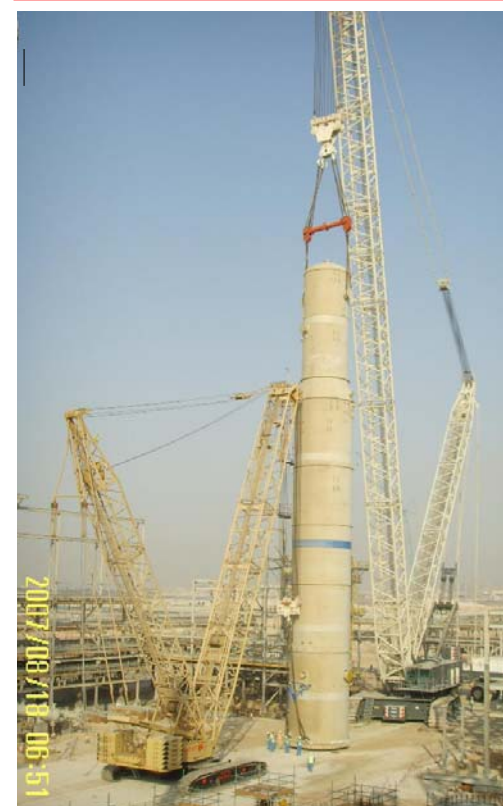
Erecting a 500 te column using a Demag CC 8800-1
