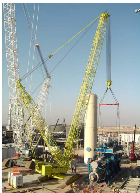
2004- Erecting a 260 te compressor in Qatar.
