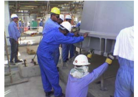
Our surveying team performs checks on foundation holding bolts and vessel orientation prior to lowering onto foundation.
