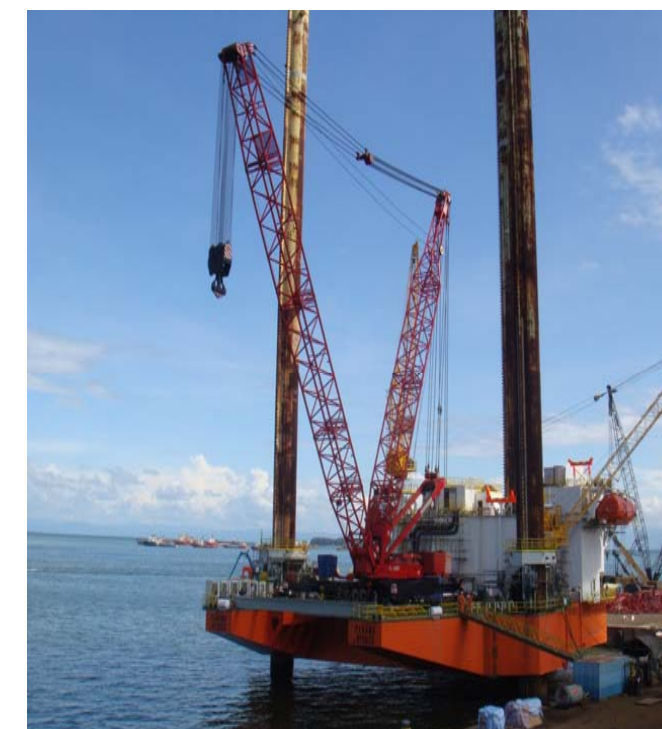
2007- 1200 te capacity crane mounted on the Global Process System Sdn Bhd jack up barge in Malaysia.
