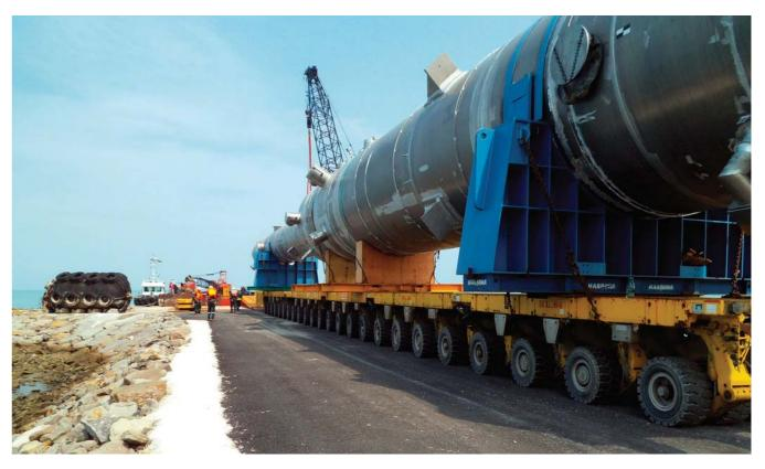
this setback AJHL's engineers proposed an alternative methodology to shift, barge and deliver the heavy equipment from storage to the project site. A carefully-scheduled SPMT delivery phase using 2 PPU and 28 axle lines ensured the equipment was delivered directly under the hook of the cranes and timed to co-ordinate with the planned lifts of all the equipment. The next phase saw the Demag CC2800-1 built into 108m SSL-LSL configuration and travel to the new flare.
