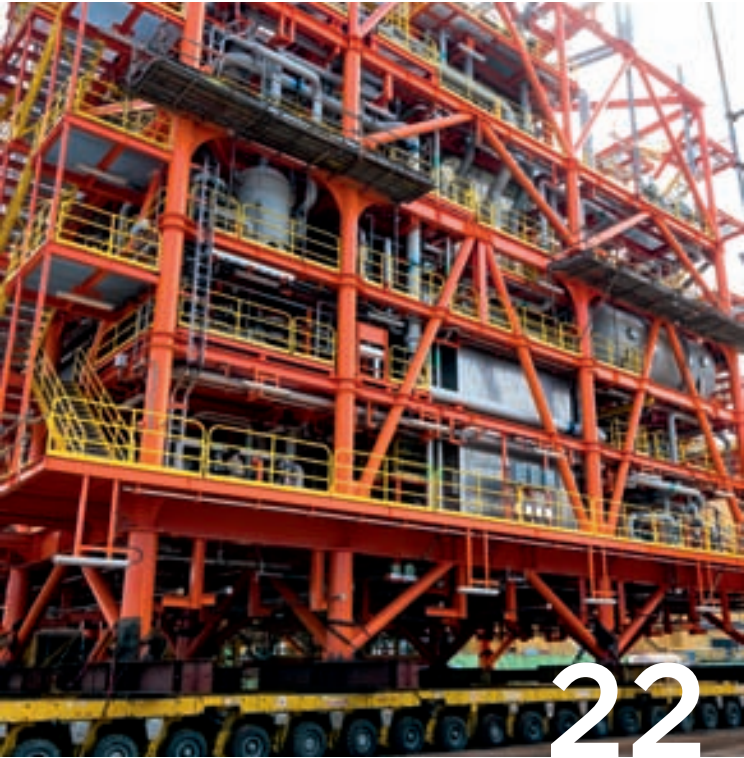
FRONT COVER IMAGE Integrated triple boiler module fabricated by Asia Offshore Services Singapore (AOS), a subsidiary of AJHL. An excellent example of the combination synergies of module fabrication, heavy lifting, heavy transportation and loadouts available within the Al Jaber Heavy Lift Group. See page 22 for story.
