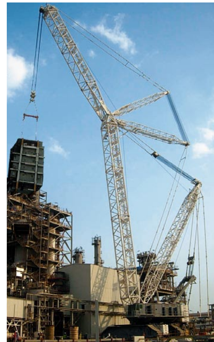
△ Installation of a 120 te boiler using a Demag CC8800 in Qatar.
