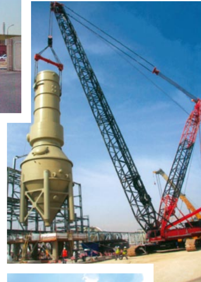
▽ Installation of a 240 te brine evaporator using a Demag CC 2500 as main crane and a Demag CC1800 as tailing crane in Qatar.
